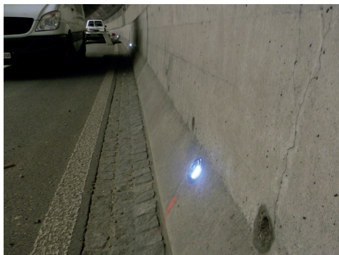
Tunnel Stephanshorn San Gallo
